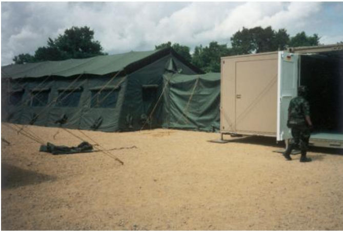
• FIG. 11.10 Vestibule connects ISO and TEMPER.
